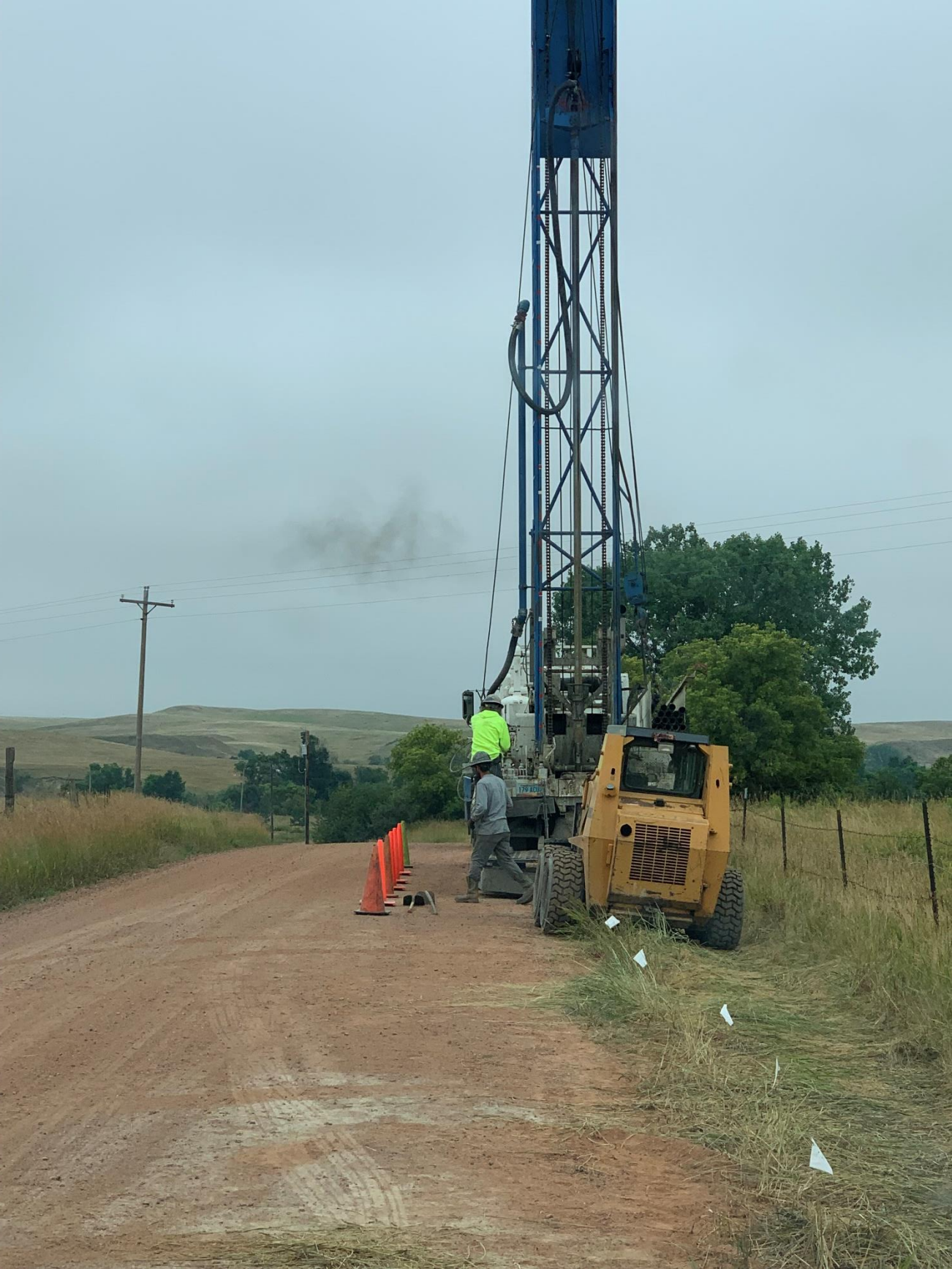
Figure 3: Drilling along Lehigh Drive
