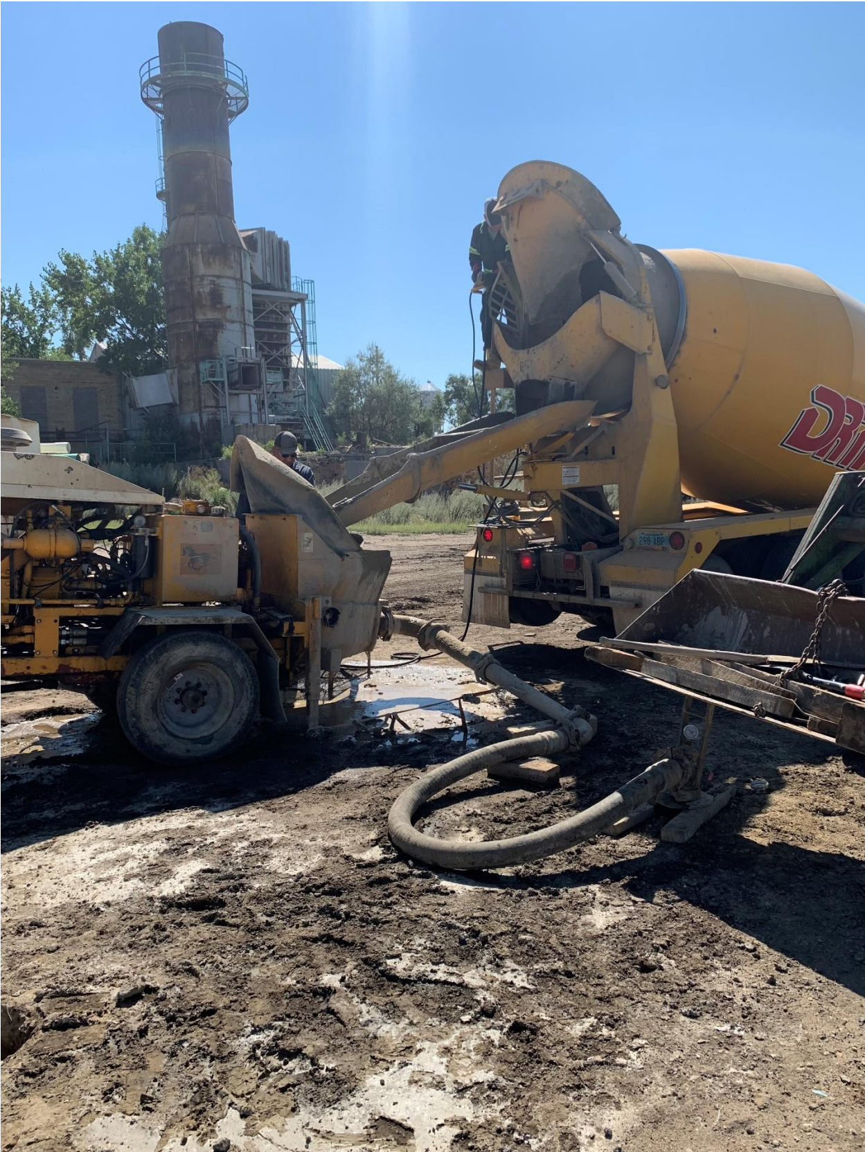
Figure 5: Pumping grout in front of the Lehigh Briquetting Plant
