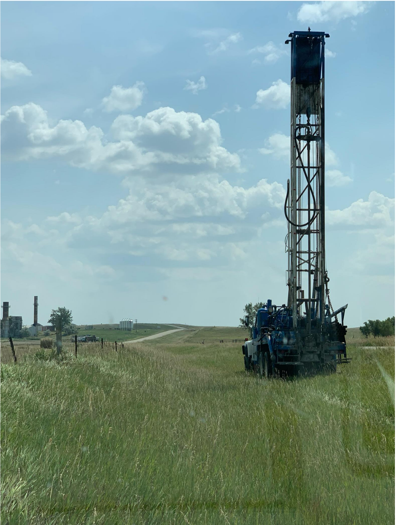
Figure 1: Drill rig setting up to drill along Lehigh Road
