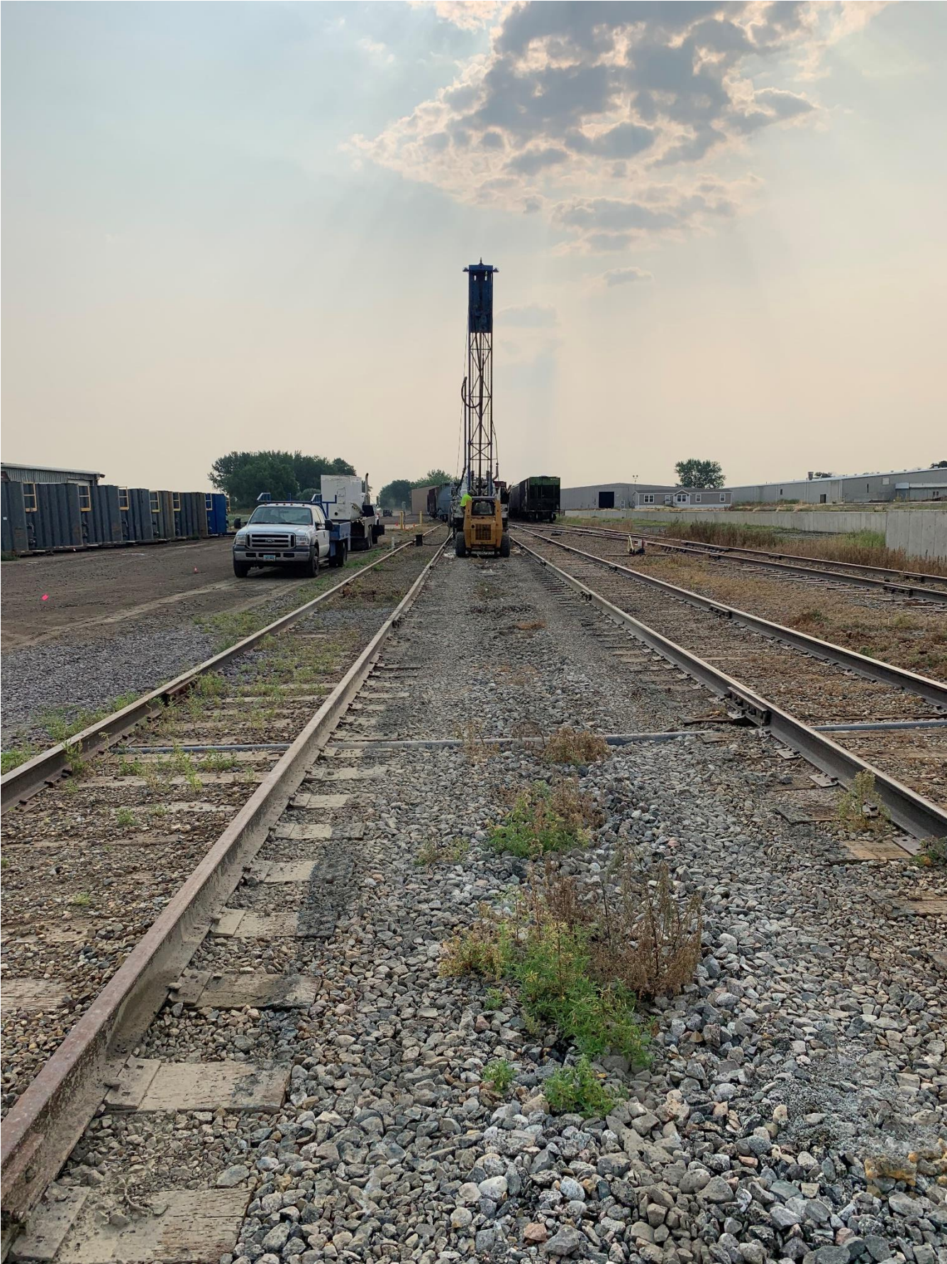
Figure 2: Drilling between railroad tracks
